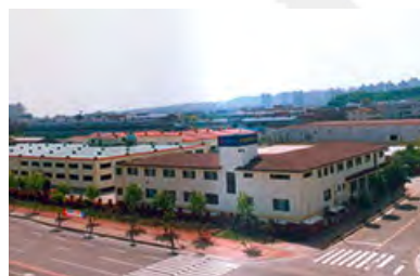
Incheon Facility (KOREA)
