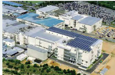
Yokaichi Facility (JAPAN)
