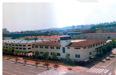
Incheon Facility (KOREA)
