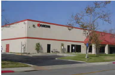
California Facility (USA)
