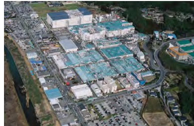
Sendai Facility (JAPAN)
