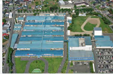
Okaya Facility (JAPAN)
