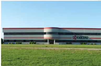
Ohio Facility (USA)
