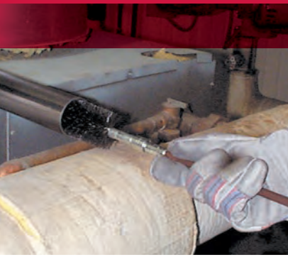
Cleaning boiler pipes with a flue brush.
