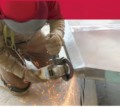
Grinding on a platform for weld preparation.
