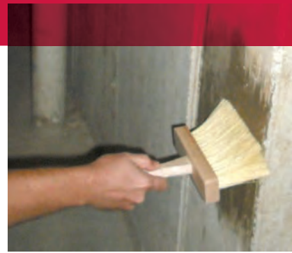
Applying waterproofing material with a masonry brush.
