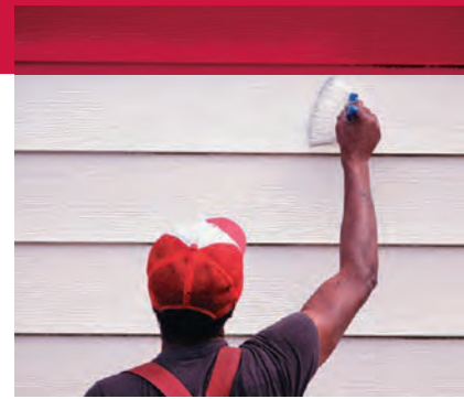
Applying paint to clap board siding.
